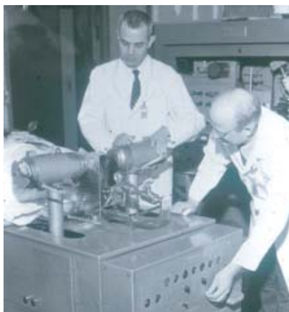
Fig.-4: First clinical positron imaging device
